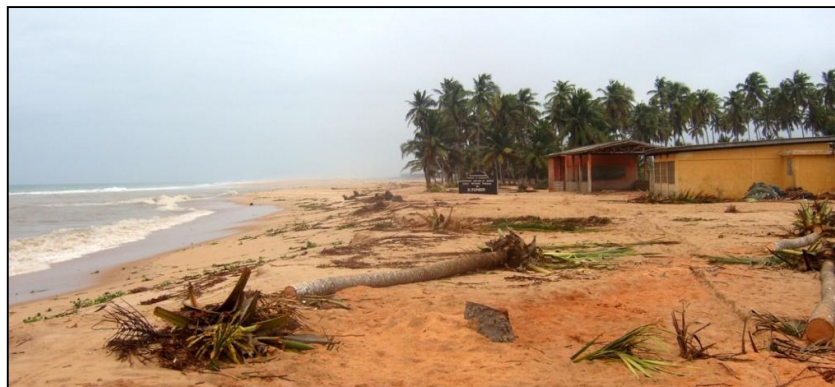
Photo 3. Photographic images showing the devastation of erosion in front of the public primary school at Djondji
